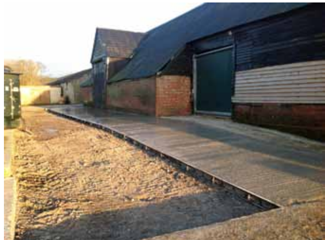
Concreting a new track
