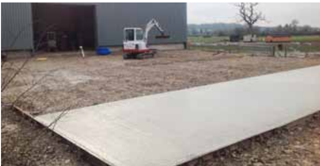
The first slab of concrete laid
